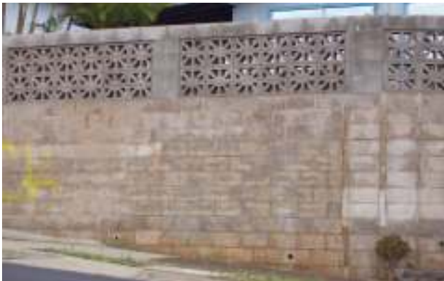
Example of cinder block wall with patterning
