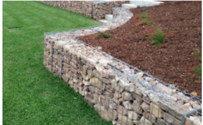
Example of gabion wall
