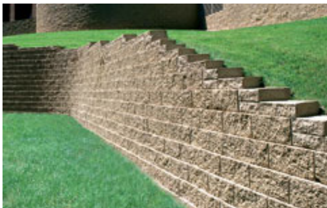
Example of terraced retaining wall
